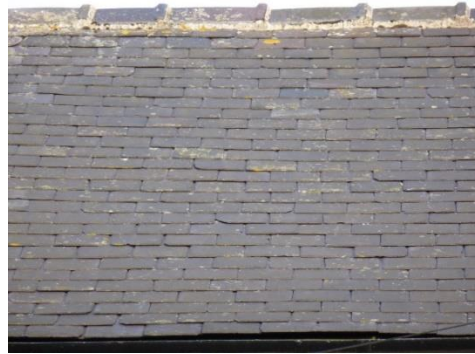
Natural slate roof
