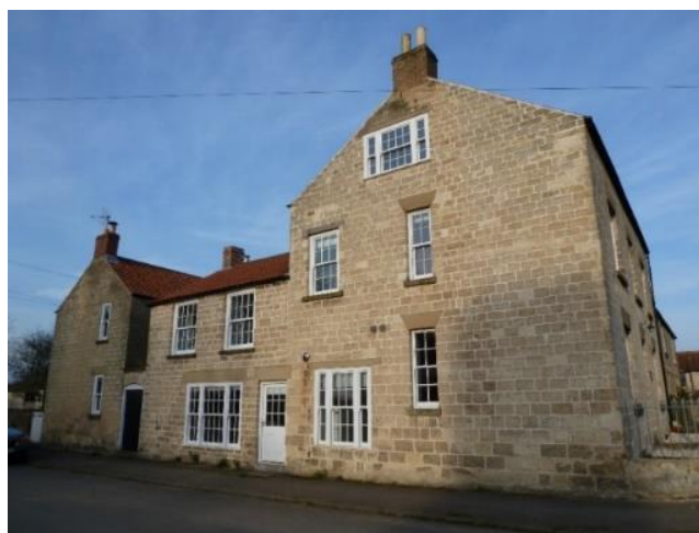
Lime pointing at Prospect House
